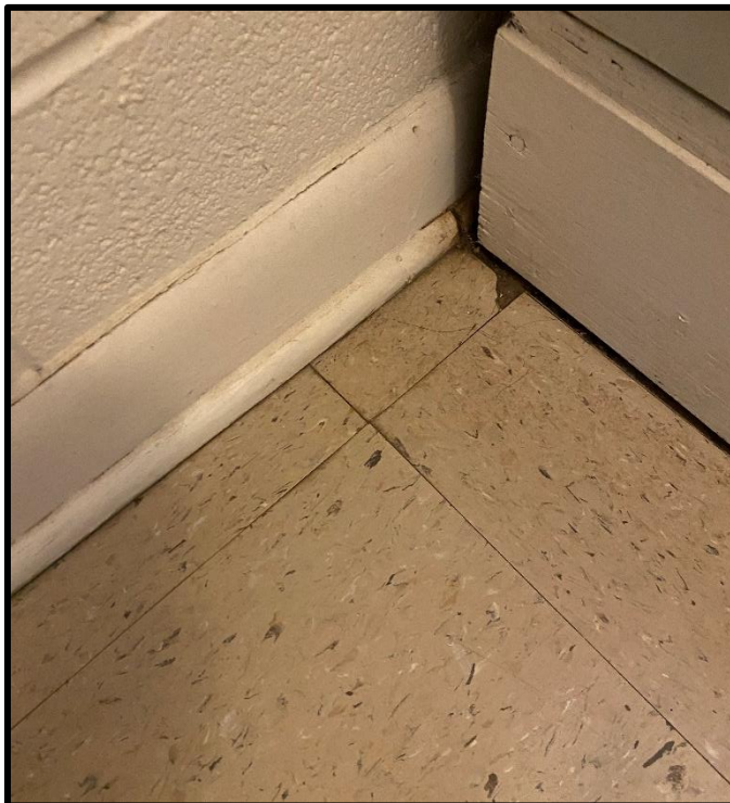
Photograph 9. ACM-9 – Floor tile in southern portion of Shower Room.
