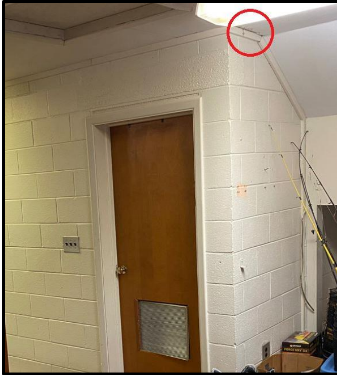
Photograph 13. ACM-13 – Ceiling plaster in southeastern portion of Level 2 Open Area.
