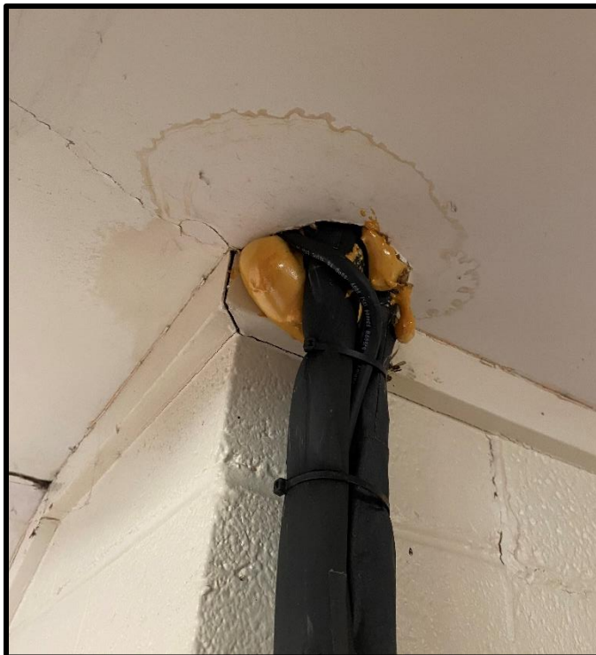
Photograph 11. ACM-11 – Conduit caulking on ceiling north of stairway in Level 2 Open Area.
