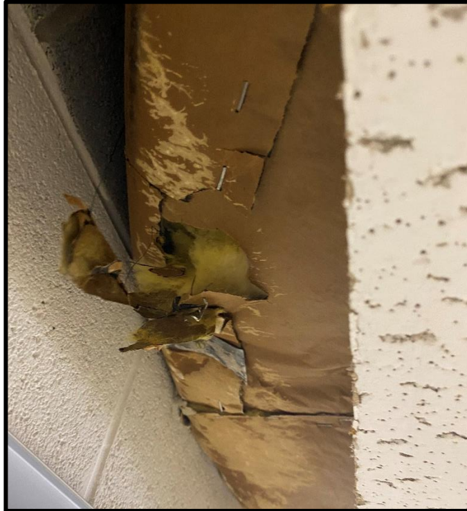
Photograph 5. ACM-5 – Ceiling insulation near western wall of central Corridor.
