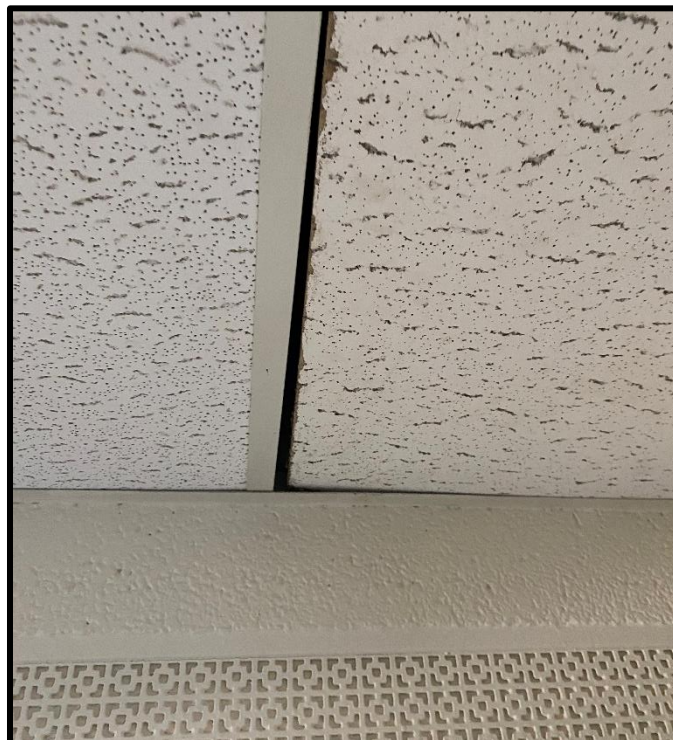
Photograph 8. ACM-8 – Ceiling tile in eastern portion of Lobby.
