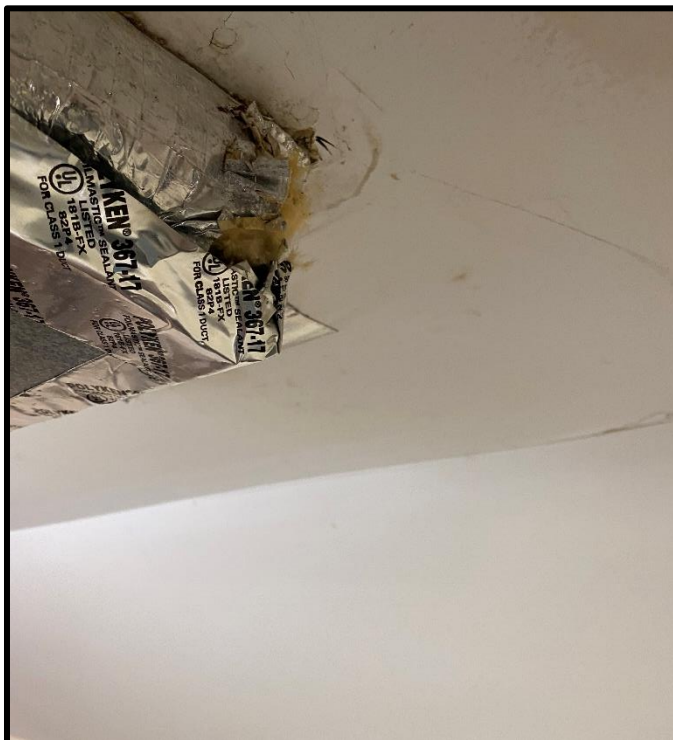
Photograph 12. ACM-12 – HVAC insulation on ceiling north of stairway in Level 2 Open Area.
