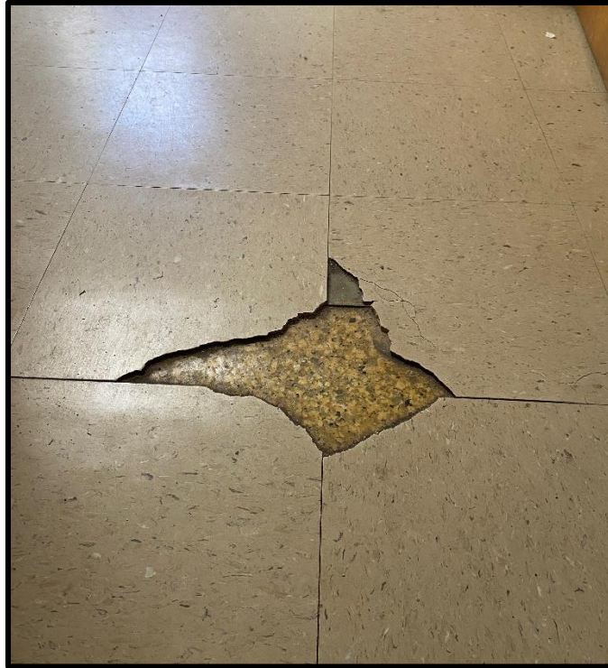
Photograph 1. ACM-1 – Floor tile in northeastern corner of Break Room.
