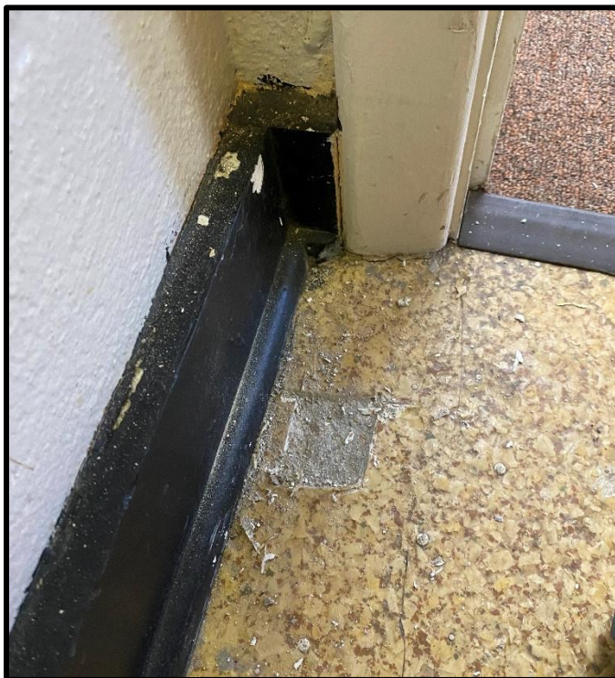
Photograph 10. ACM-10 – Level 1 Stairway floor linoleum near western wall before stairway.
