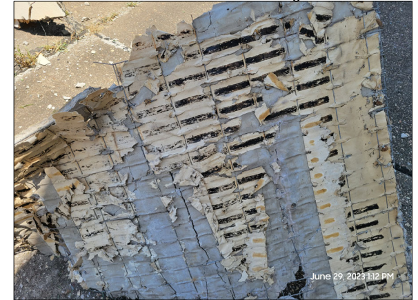
EXTERIOR MATERIAL , PAPER, 2X2, METAL WIRE GRID, 1" OF GYPSUM MATERIAL, AND SEVERAL LAYERS OF PAINT.
