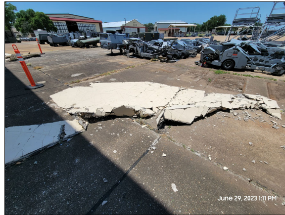
SECTION OF WALL FROM STORM
