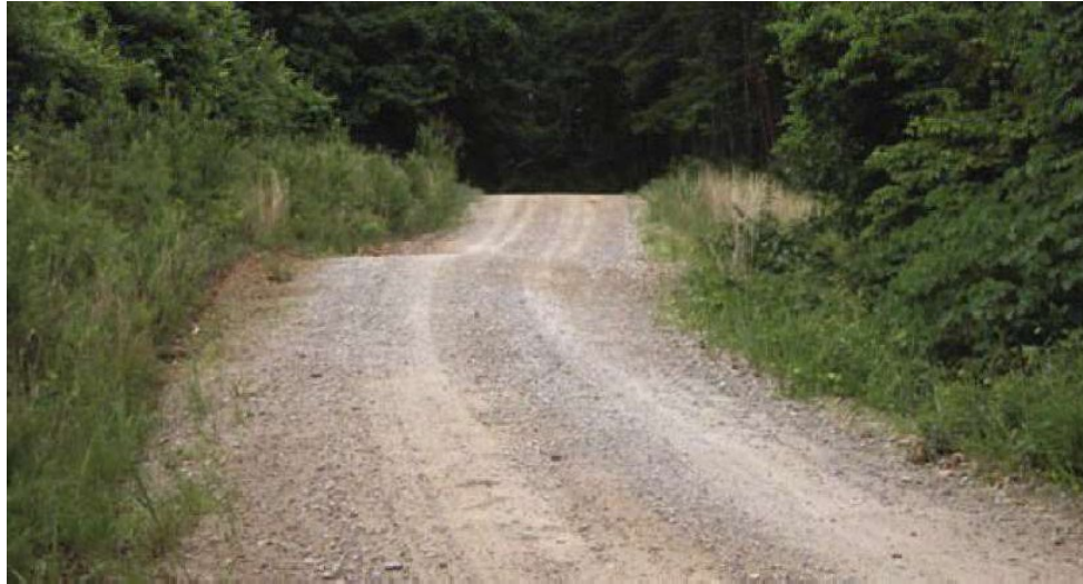
Figure 02: Example #2 Maintenance Level 3 Road
