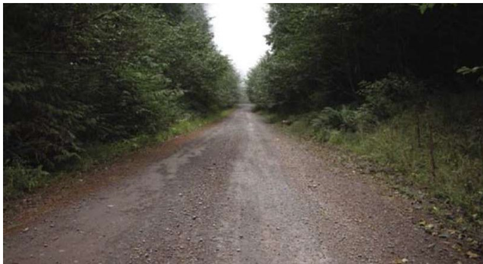
Figure 01: Example #1 Maintenance Level 3 Road
