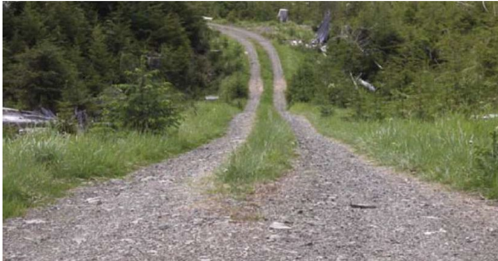
Figure 03: Example #3 Maintenance Level 3 Road
