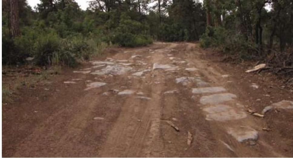
Figure 04: Example #1 Maintenance Level 2 Road
