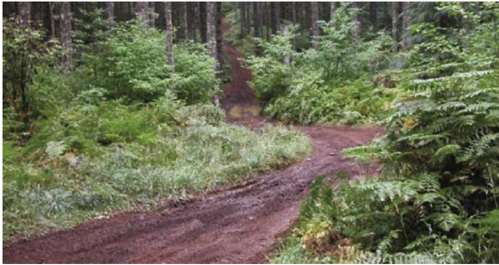
Figure 05: Example #2 Maintenance Level 2 Road
