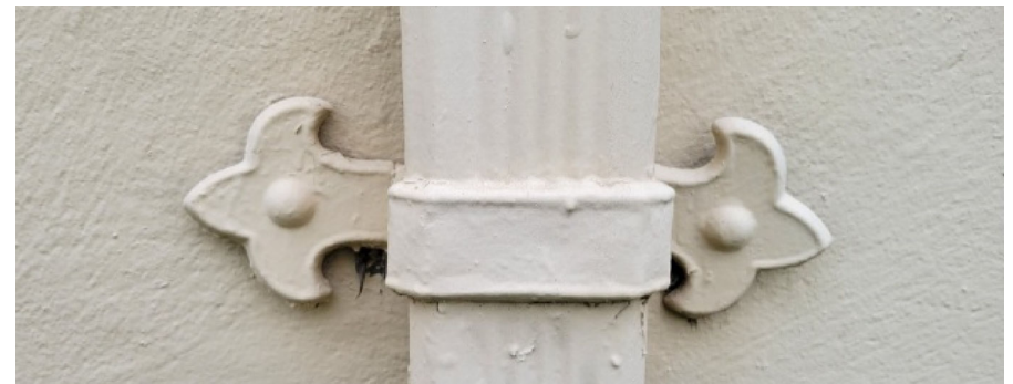
REFERENCE ONLY - DOWNSPOUT BRACKET.
