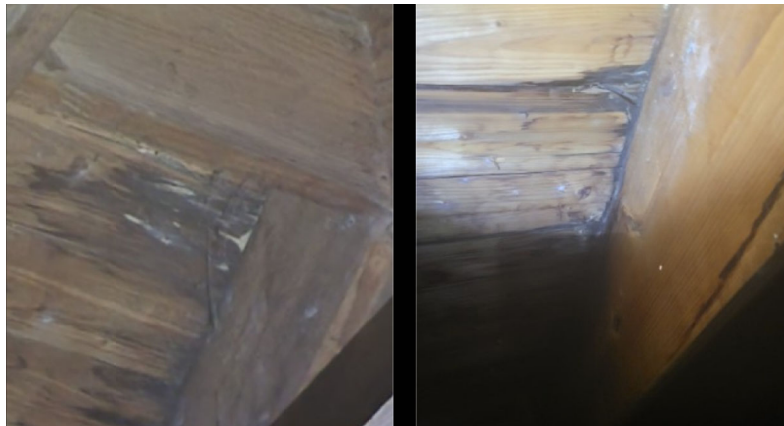
EXAMPLE OF RAFTER & DECKING TO BE REPAIRED
