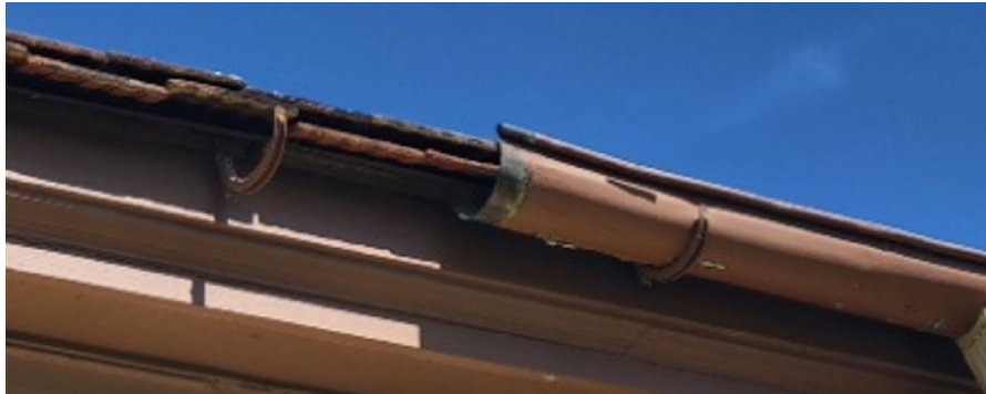
EXISTING GUTTER SYSTEM
