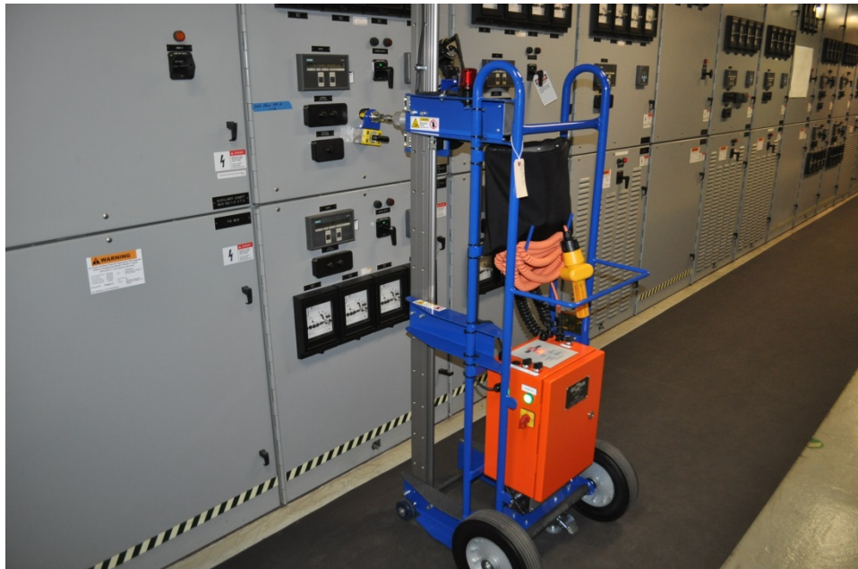
Figure 1. Remote Racking Mechanism
