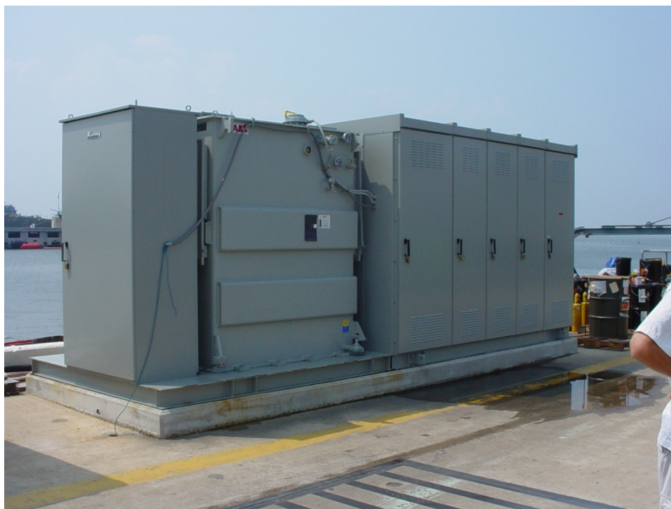
Figure 12-5. Skid-Mounted Substation with Single-Pole Connections
