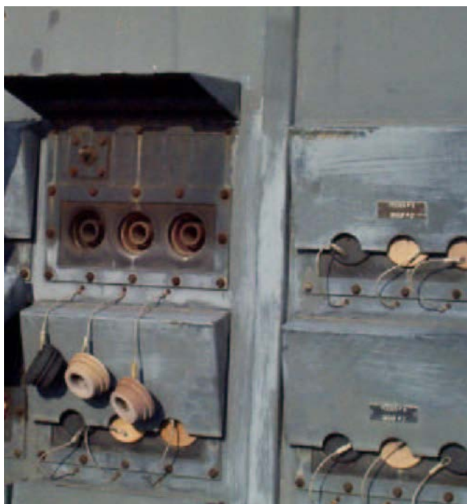
Figure 12-5. Skid-Mounted Substation with Single-Pole Connections
