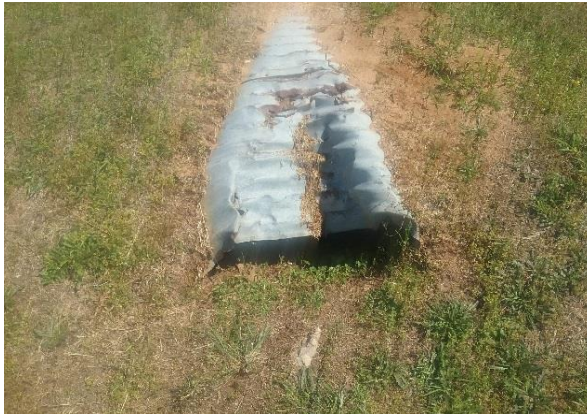
Figure 31: Crushed Pipe
