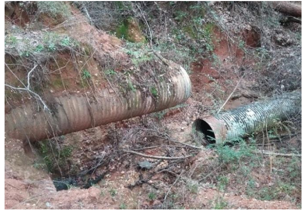
Figure 32: Broken Pipe
