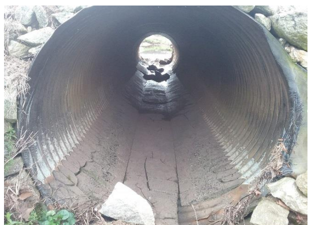
Figure 30: Missing Coating
