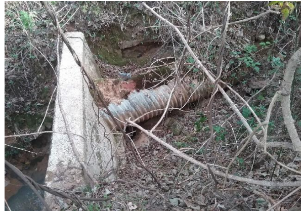
Figure 34: Damaged Headwall
