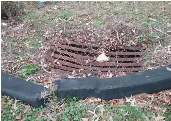
Figure 33: Damaged Grate
