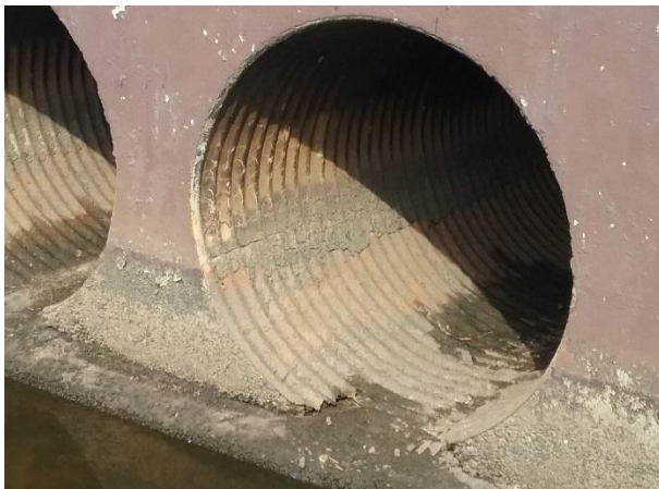
Figure 29: Rusted Invert
