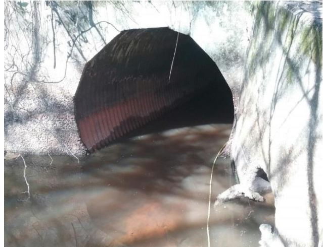
Figure 18: Rusted CMP
