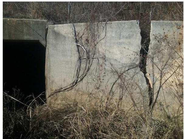
Figure 22: Cracked Headwall
