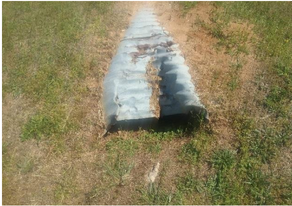
Figure 31: Crushed Pipe
