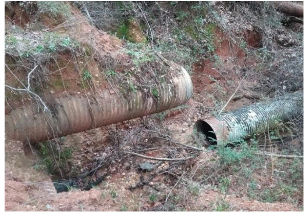
Figure 32: Broken Pipe
