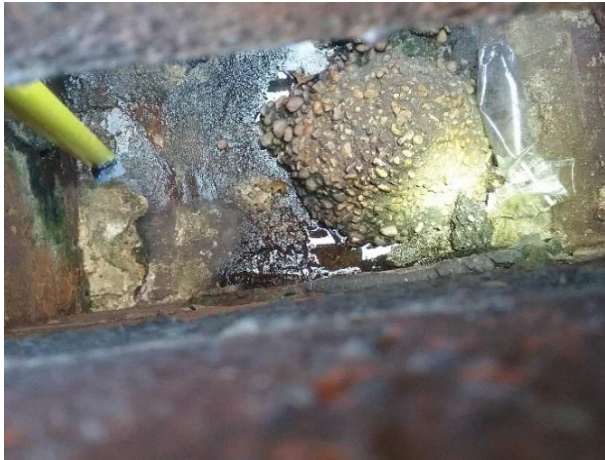
Figure 27: Concrete Deposits
