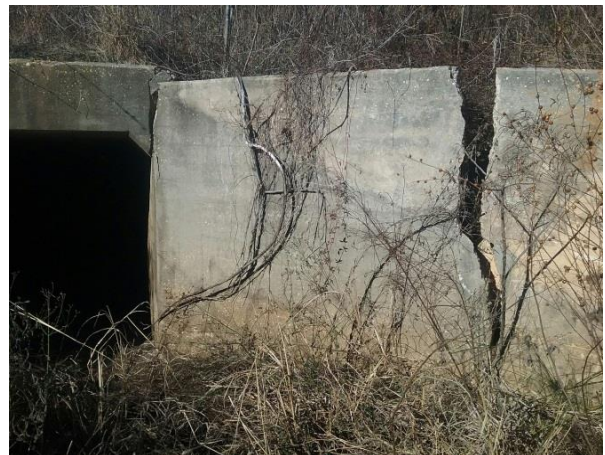
Figure 22: Cracked Headwall
