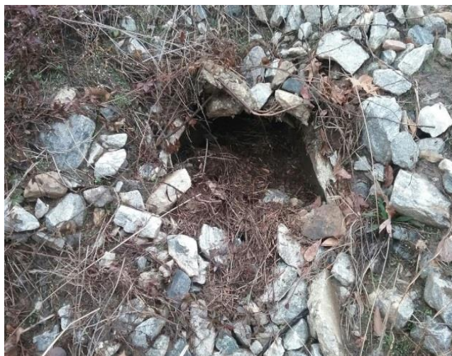
Figure 19: Defective Headwall
